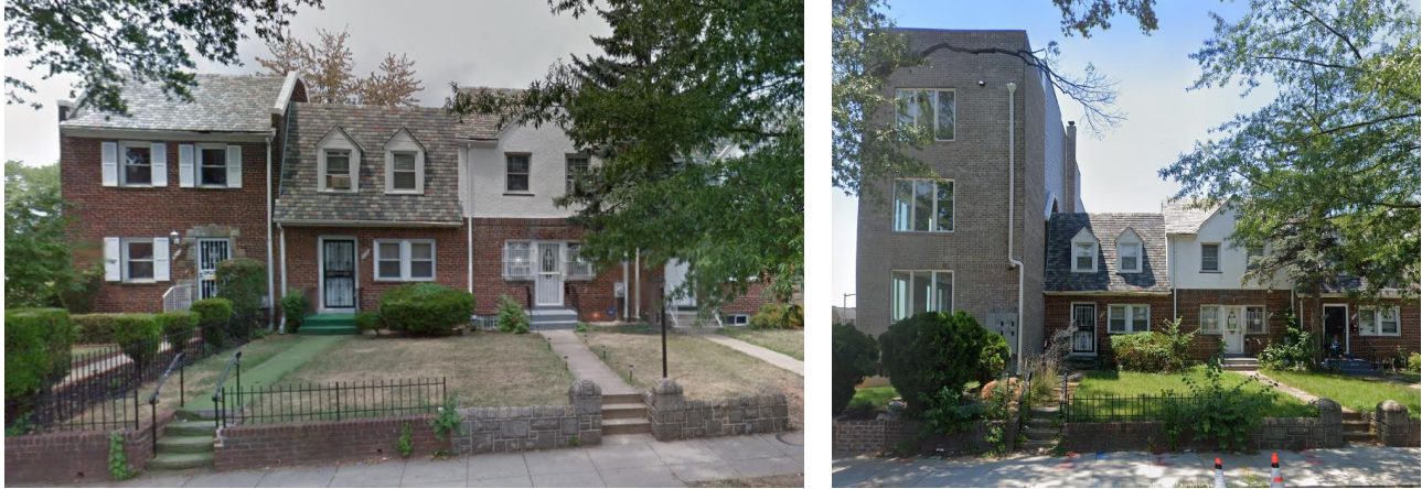
Figure 2. Before and after comparison of a recent apartment house conversion from a semi-detached single-family house.
